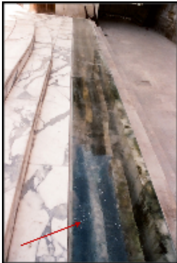
Fig.3 Shows the dense layers of biological colonization accumulated on the surface of the water duct. The arrow point to the water drops condensed on the glass surface.
